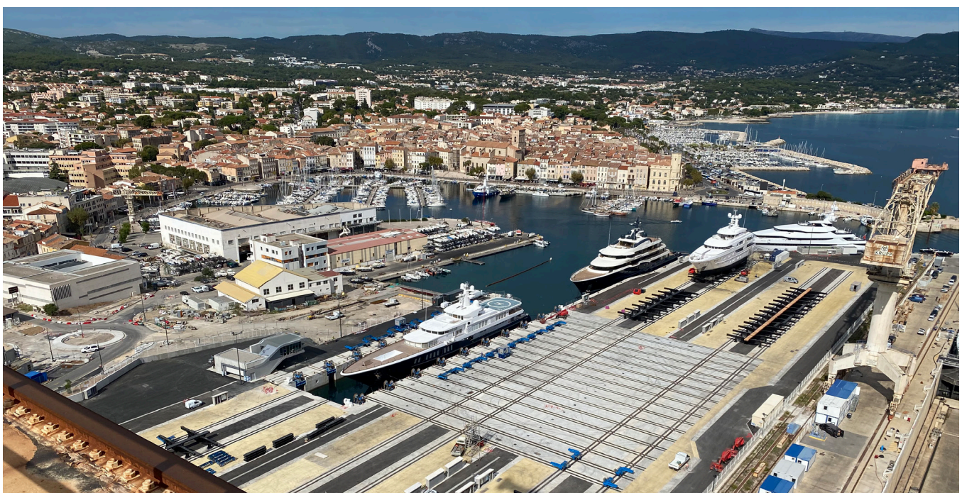
This yard can service up to six yachts simultaneously with the OmniLift and Transfer system
